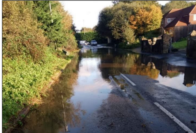
Photograph showing Frog Grove Lane/Aldershot Road flooding – October 2021. The footpath is impassable, and the water in the centre of the highway was too deep for pedestrians or cyclists, and some vehicles.
