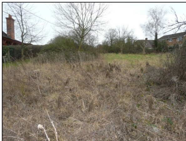
Site of the community car park prior to works commencing - Land to the west of Wood Street Infant School
