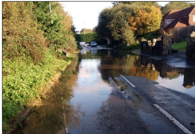
Photograph showing Frog Grove Lane/Aldershot Road flooding – October 2021. The footpath is impassable, and the water in the centre of the highway was too deep for pedestrians or cyclists, and some vehicles.
