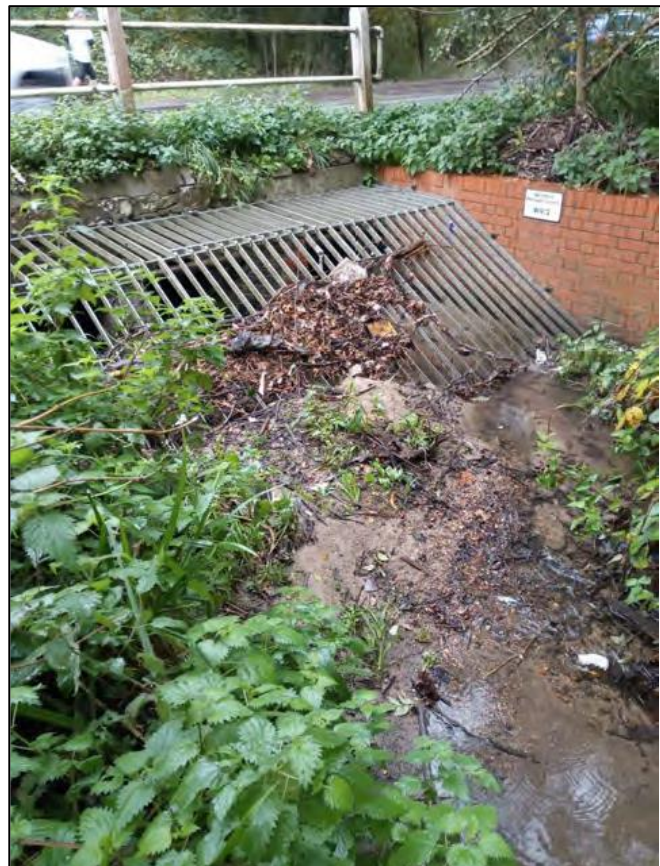
This October 2021 photo shows a grille after the Head Groundsman from Worplesdon Parish Council removed all of the debris that had blocked the flow of water through it, plus he had also dragged a double mattress out of the flow.
