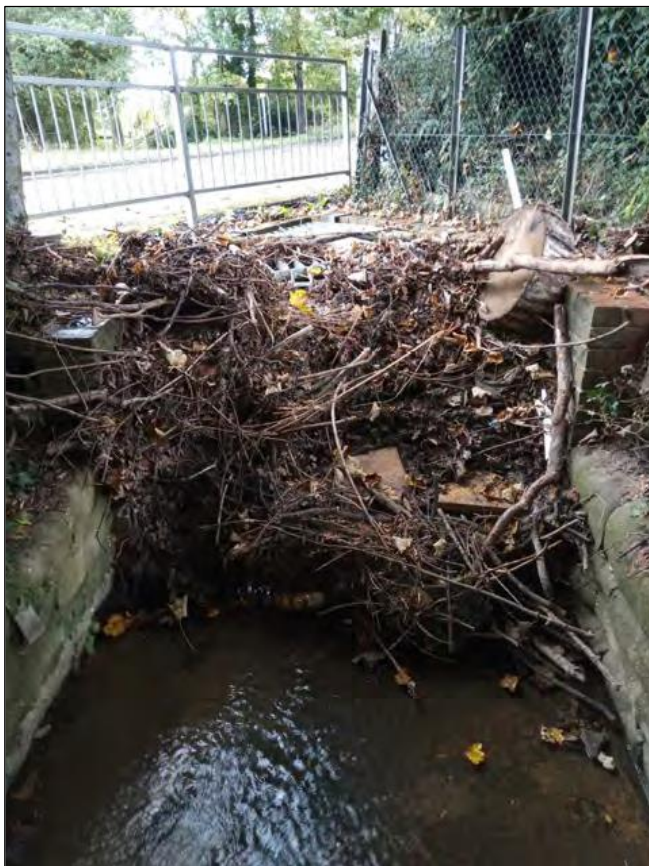
This October 2021 photo shows a grille after the Head Groundsman from Worplesdon Parish Council removed all of the debris that had blocked the flow of water through it, plus he had also dragged a double mattress out of the flow.
