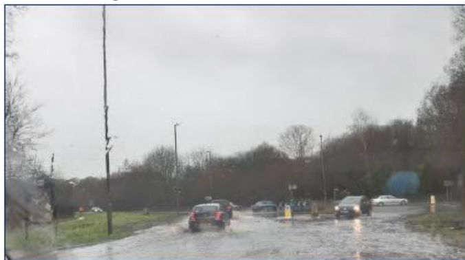
Photograph showing Woking Road/Salt Box Road flooding – Spring 2020
