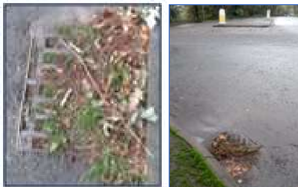
Photos show the packed drains on Holly Lane and on the upper roundabout
