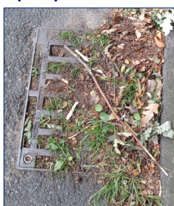
Photo showing the packed debris blocking the drain on Holly Lane.
