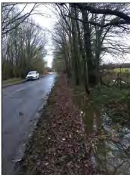
Photographs showing the issue the blocked ditch at Gravetts Lane is causing (January 2020). This is after the water had receded over the course of a weekend.
