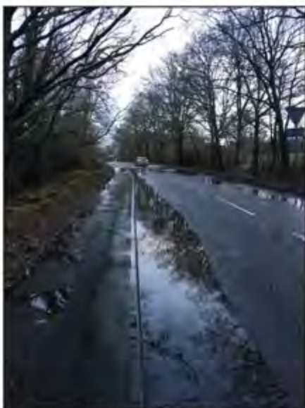
Photographs showing the issue the blocked ditch at Gravetts Lane is causing (January 2020). This is after the water had receded over the course of a weekend.
