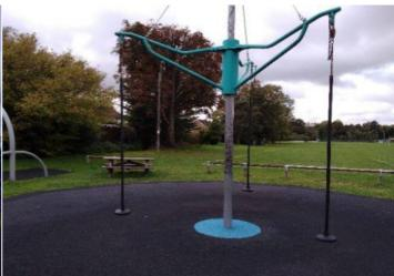
Finding: This item of equipment relies on a single post, or a Action: Ensure that regular detailed inspections are line of posts, for stability and extra care needs to be taken with equipment of this nature to avoid the potential for catastrophic failure
