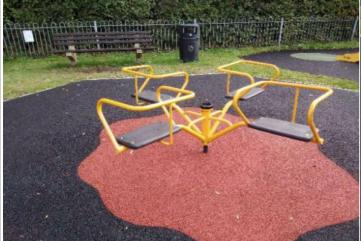
**Finding:** Parts of the steel structure protrude beyond the protected elements of the seat and fail to meet the requirements of BS EN 1176:2008 Part 5
