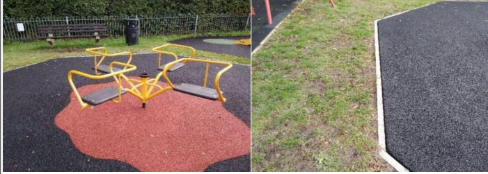
**Finding:** There are gaps opening between the surfacing and **Action:** Monitor for any further deterioration and repair as the edging surround or between the joints in the surfacing required
