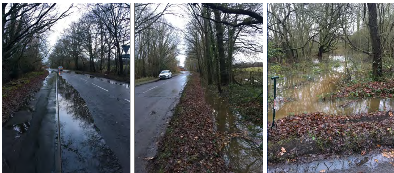
Photographs showing the issue the blocked ditch at Gravetts Lane is causing (January 2020). This is after the water had receded over the course of a weekend.
