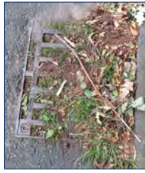
Photo showing the packed debris blocking the drain on Holly Lane.
