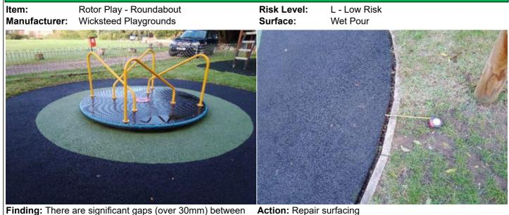
**Finding:** There are significant gaps (over 30mm) between the surface and the edging or between the joints in the surface; these are large enough for a small foot to enter
